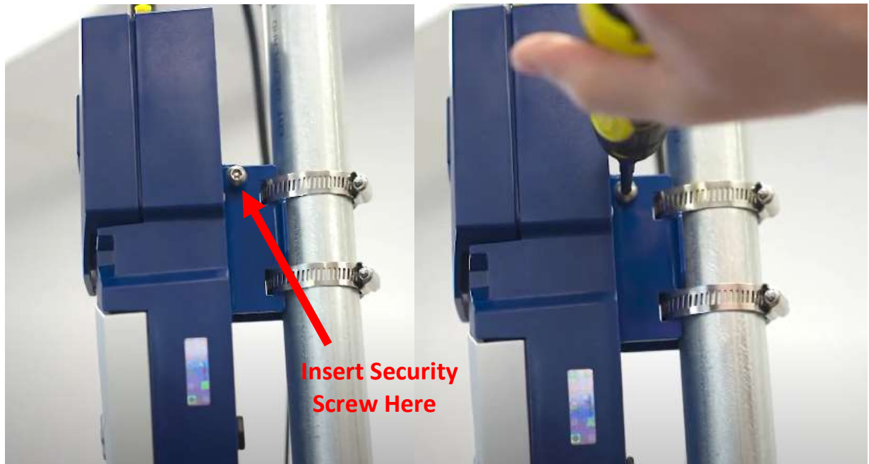
Figure 13: Installation of security screw
